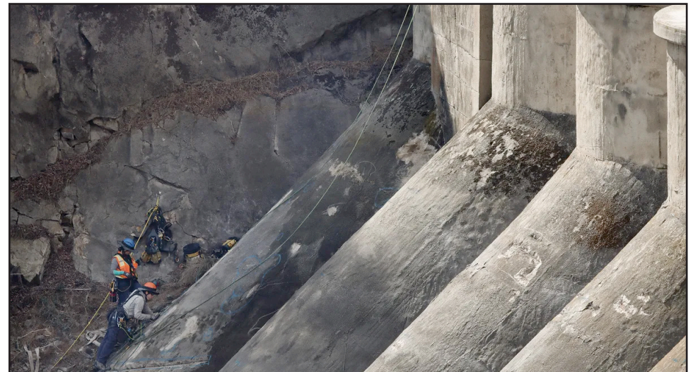
More than 100 years old, San Diego's Lake Hodges Dam is one of 42 dams where the state has restricted storage because of safety concerns. Repairs began in 2022 and the dam is expected to be replaced by 2034. Photo by John Gastaldo for CalMatters
